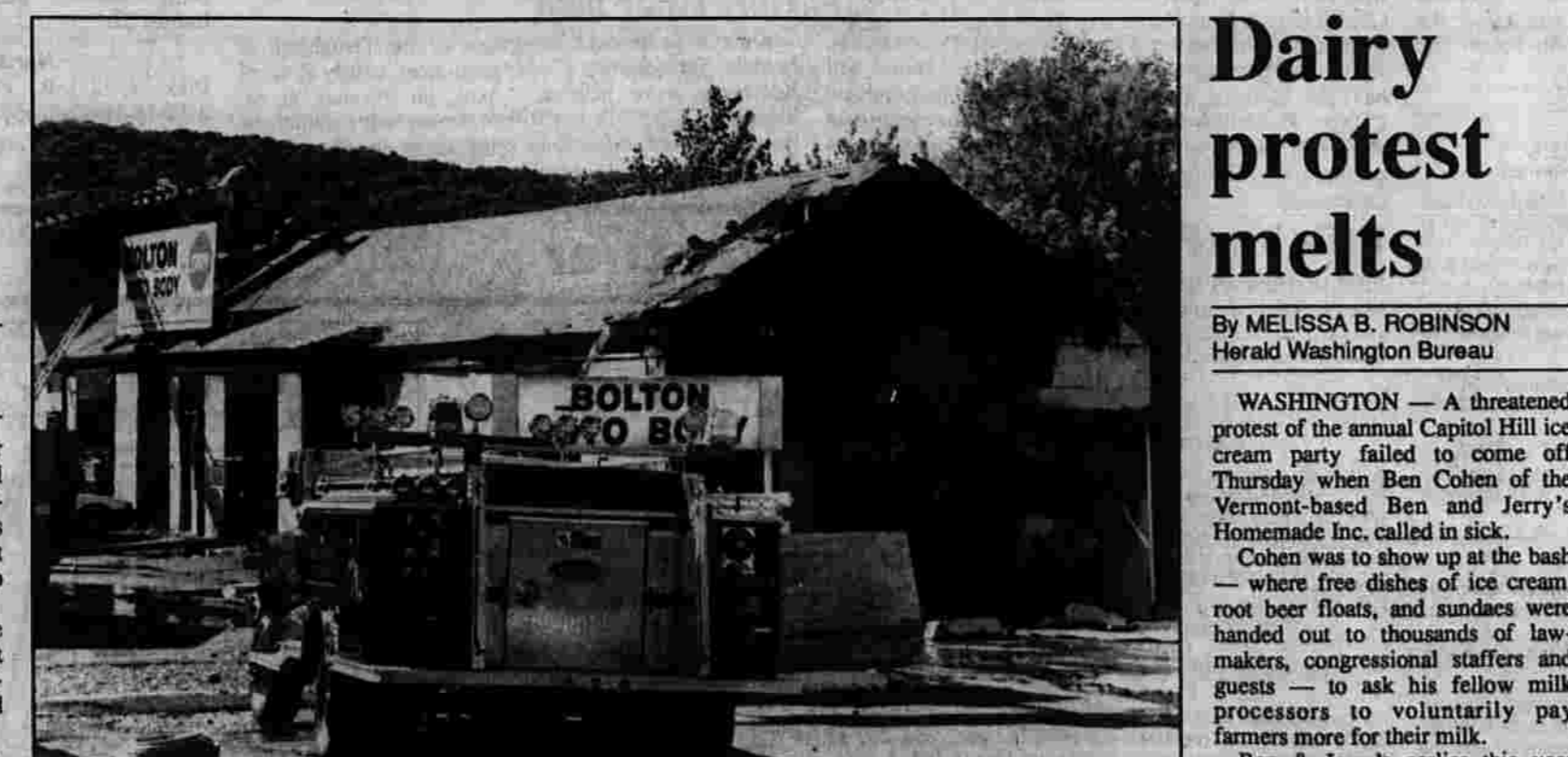
BUILDING DESTROYED - Volunteer firefighters from Bolton and several surrounding towns rebuilt the aftermath of a three-hour blaze at the Bolton Auto Body shop on Route 6 Friday. The fire destroyed the interior of the building. There were no injuries. Please see FIRE, page 6.
